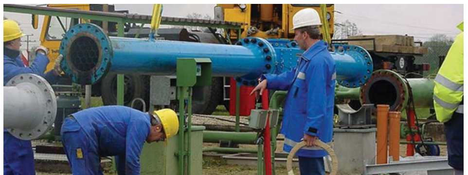
KROHNE Oil & Gas engineering supervising installation of custody-transfer metering system, later to be included in leak detection system
